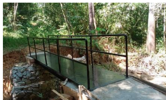
Figure 2 – Reconstructed bridge completed.
